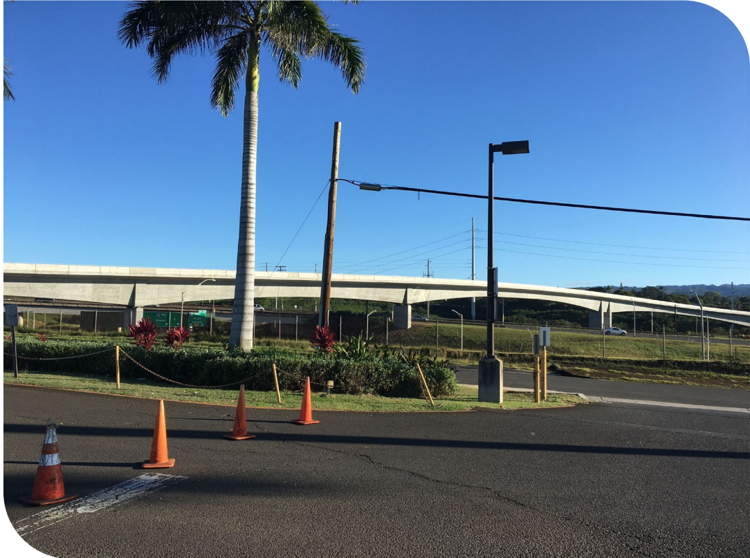
Bridge in Hawaii, part of the Honolulu Metro Rail system – outfitted with 3 Hyperion systems connected to 153 sensors for structural monitoring
